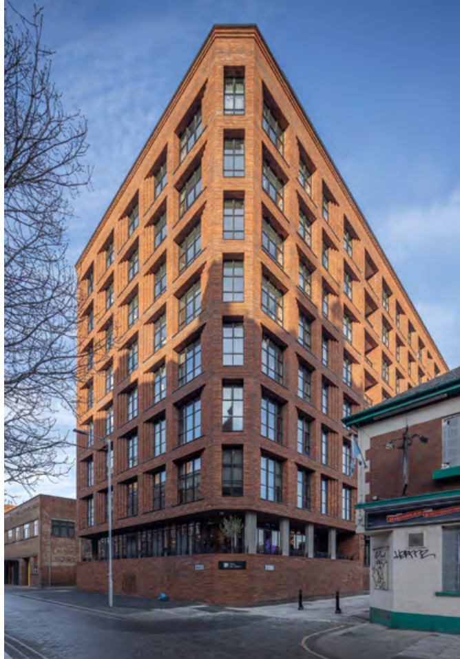
Bengal Street (One Silk St.) Development, Manchester, Marea Britanie. Sisteme utilizate: MB-59S, MB-Slimline, MB-SR50N
