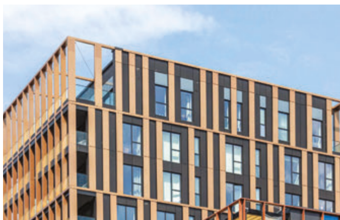
E1 Dublin Landings, Irlanda. Sisteme aplicate: MB-77HS, MB-Slide, MB-SR50N, MB-SR50N EFEKT, MB-SR50N IW
